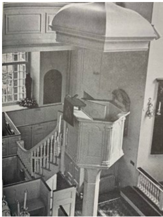
The wine glass pulpit. It is raised to give those in the box pews a better view of the preacher.
